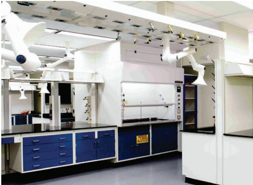
Figure 7.8a: Combination Fixed-Suspended Casework with Overhead Service Carrier
