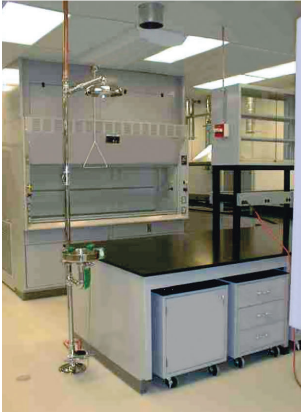
Figure 7.4b: Fixed Metal Casework with Movable Cabinetry Under
