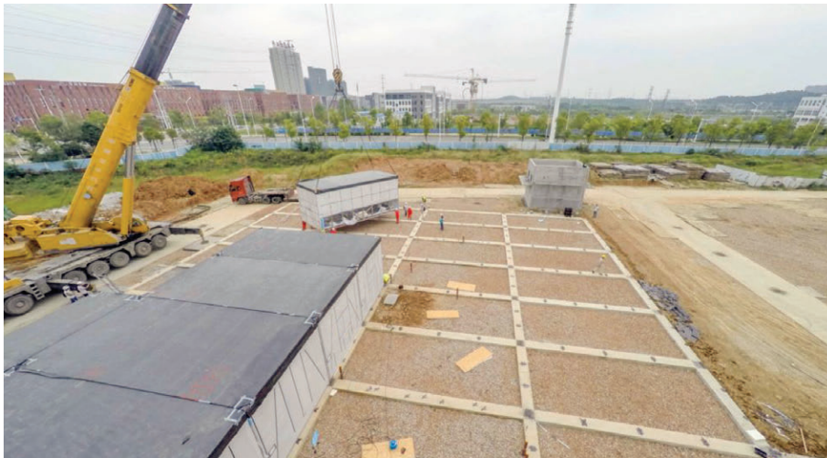
Figure 2.12: Example of Site with Modules Installed
