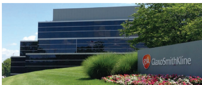
Figure 9.5: GlaxoSmithKline's Multi-Product Clinical Manufacturing Facility in Upper Merion, PA
